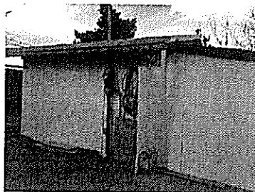
south side storage shed
